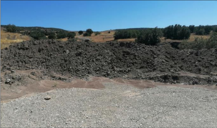
Figure 4.6. Topsoil Stored at Gaziemir-2 Location
